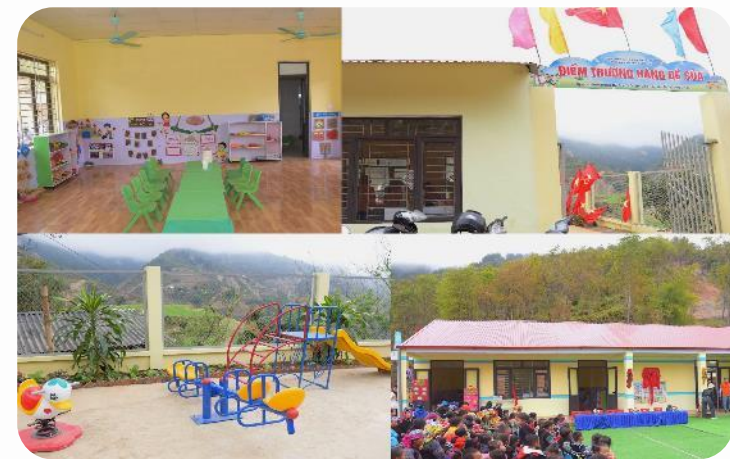
The newly constructed school provides a spacious and modern environment for preschool children.
