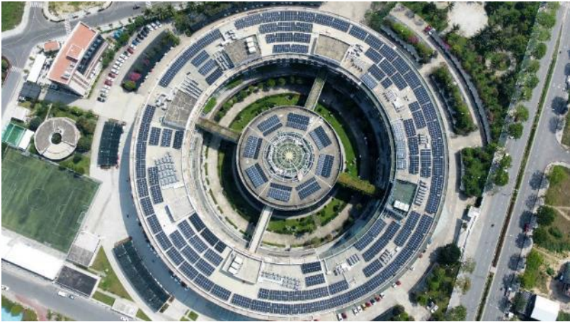
Solar energy system fully installed on the rooftop of F-Complex in Danang (Q1/2025).
